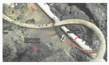
If pressure had been applied to the potable sleeve for the cutoff valve (shown above), the pipe below could shift at a gasketed connection resulting in a small leak and any intrusion could be many yards away.
