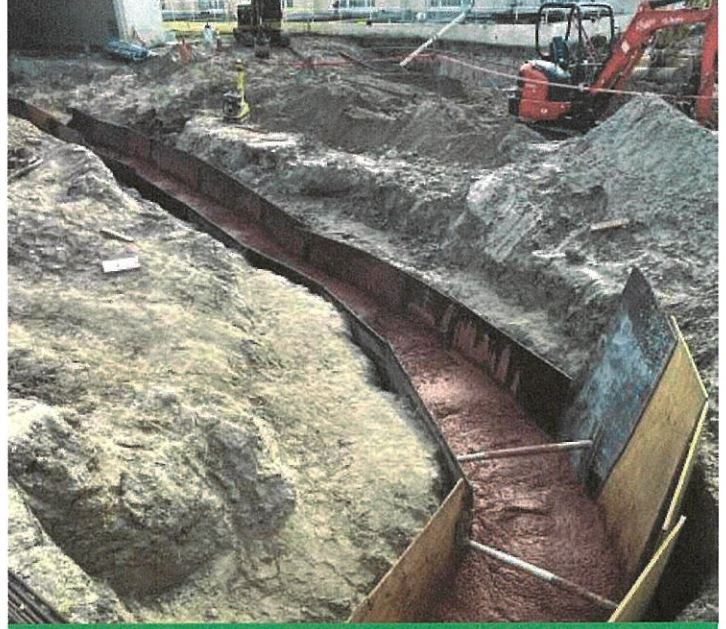
Electrical Duct Bank to Chem Building
